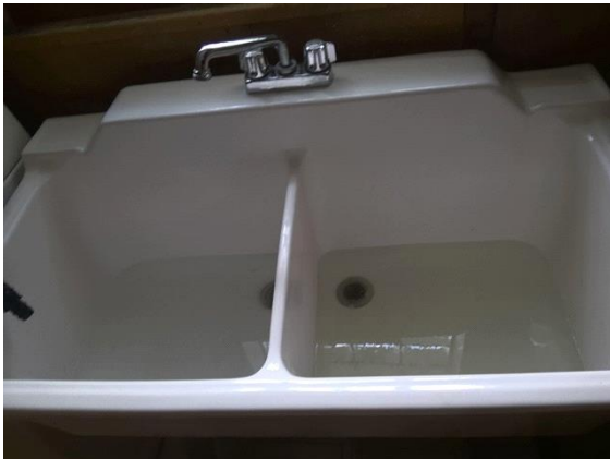
Laundry Facilities: filling writher side fills other side
